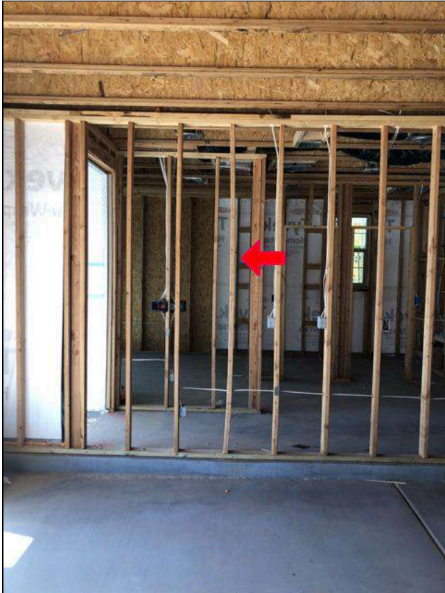
5.1 Item 1(Picture) Garage
