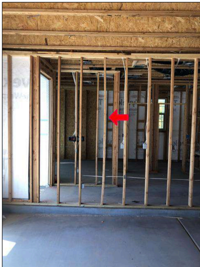
5.1 Item 1(Picture) Garage
