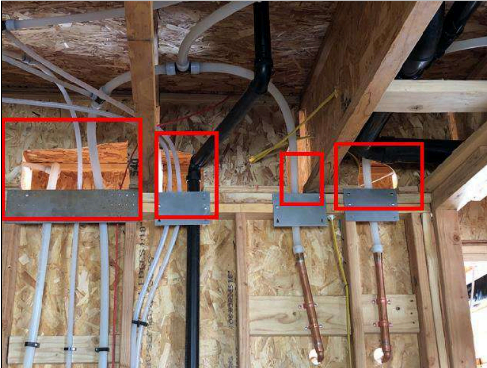
5.3 Item 1(Picture) Kitchen area
